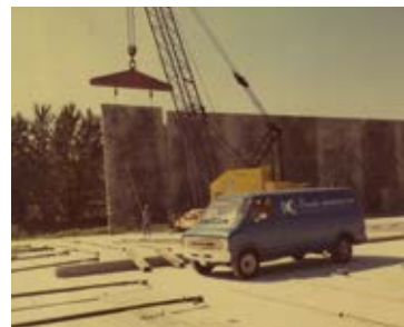
Innovative tilt-up industrial construction method / 1960s
